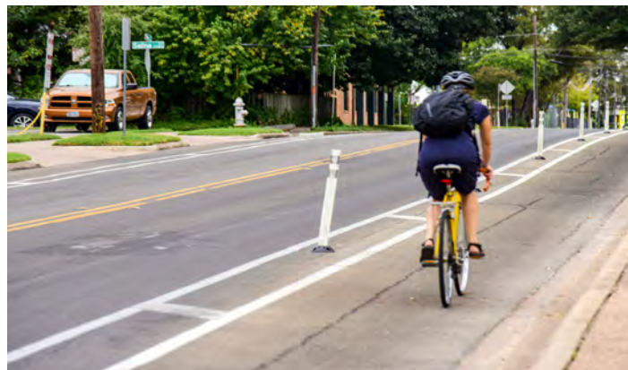
A separated bike lane with flexible posts provides dedicated space for cyclists on in Austin, Texas—an example of midblock bikeway design aimed at improving safety and comfort for riders.
